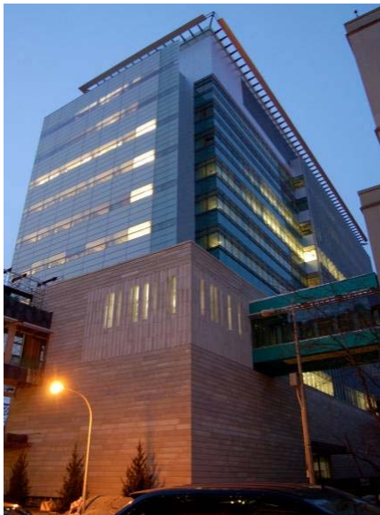
The University of Chicago Gwen and Jules Knapp Center for Biomedical Discovery Chicago, IL
